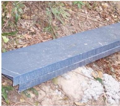
\* Double flashing – manufactured from colour matched colourbond.
